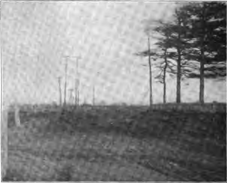
Moorestown and Masonville road, Burlington Co., before improvement.
